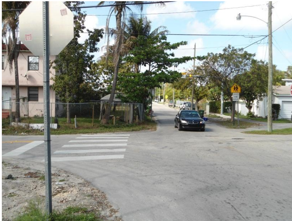
Crosswalk without access ramps and paved sidewalks
