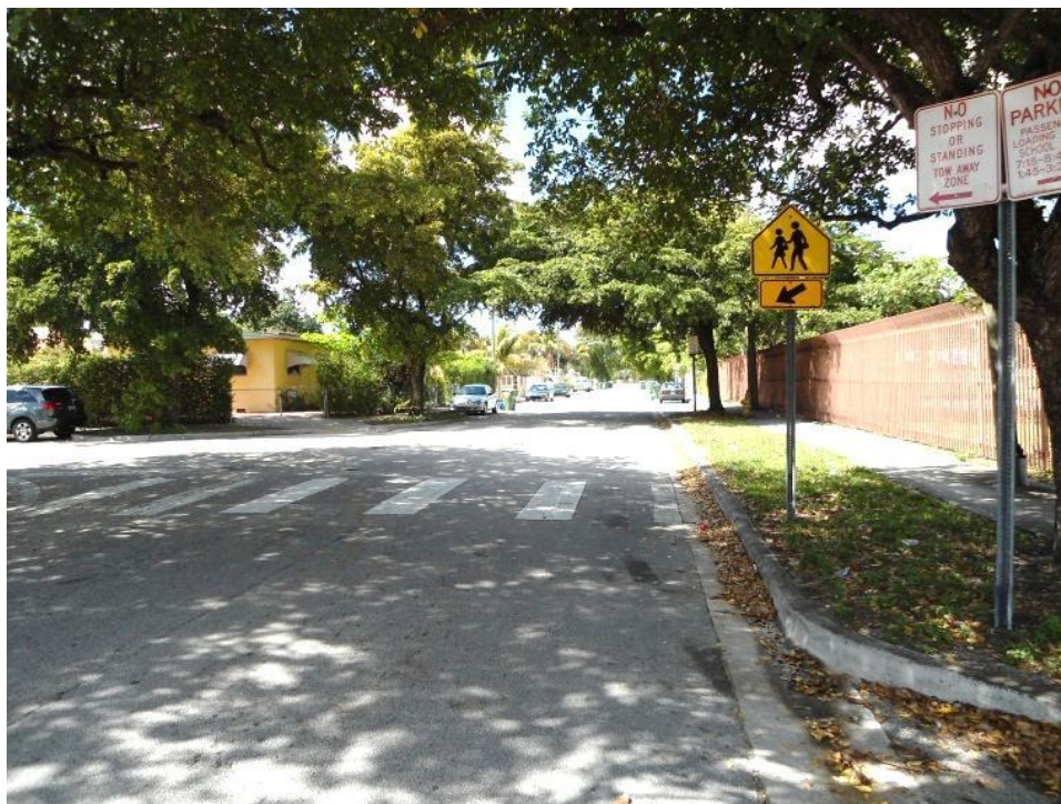
Crosswalk without access ramps and detectable warning pads
