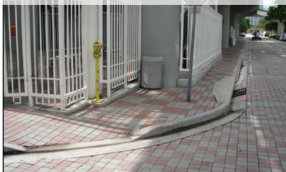
Figure 40: Fence reducing space at intersection corner
