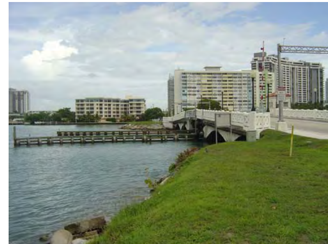
Low bridge (9' Clearance) over the Miami Beach Channel
