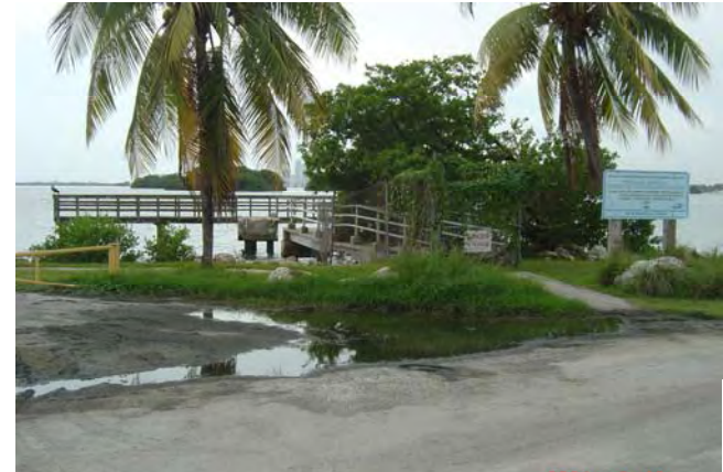
Existing dock at Pelican Harbor Park on the Kennedy Causeway
