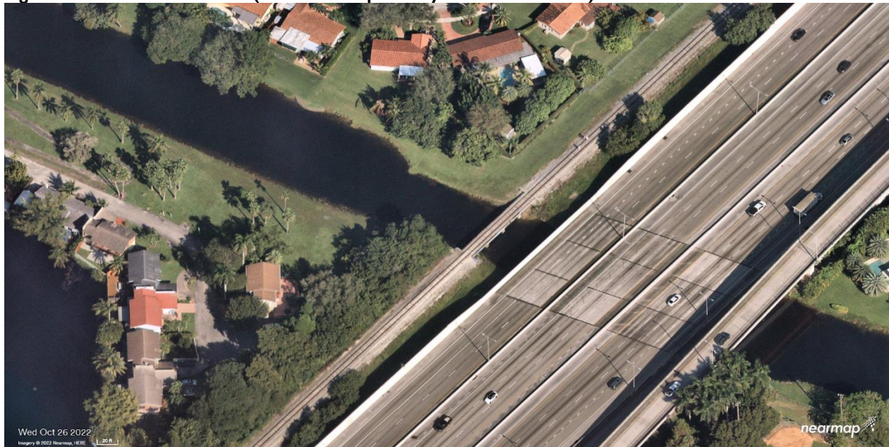
Figure 10 – Wooden Structure (Don Shula Expressway & SW 83rd Street)
