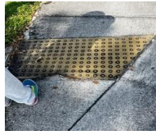
Site Visit at the Opa-locka Station
