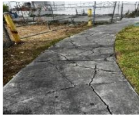
Site Visit at the Hialeah Market Station
