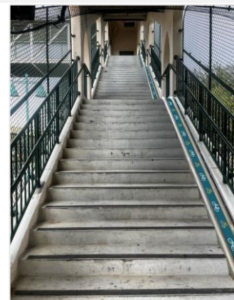
Bicycle Access Ramp
