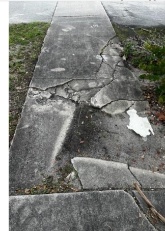
Sidewalks at the Sunshine Industrial Park have cracks
