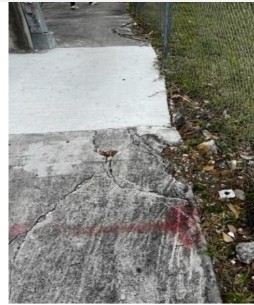
Cracked sidewalk
