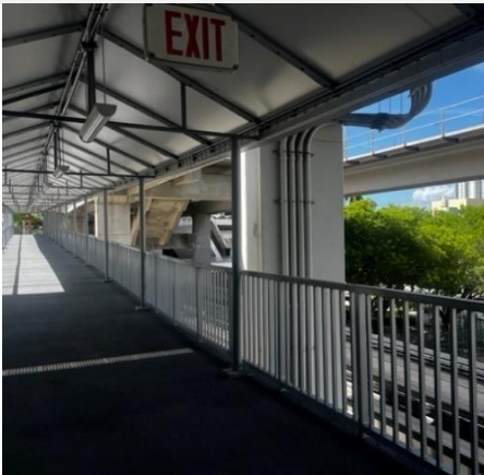
Pathway to the Government Center Metrorail Station
