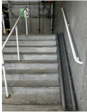
Stair access ramp in garage
