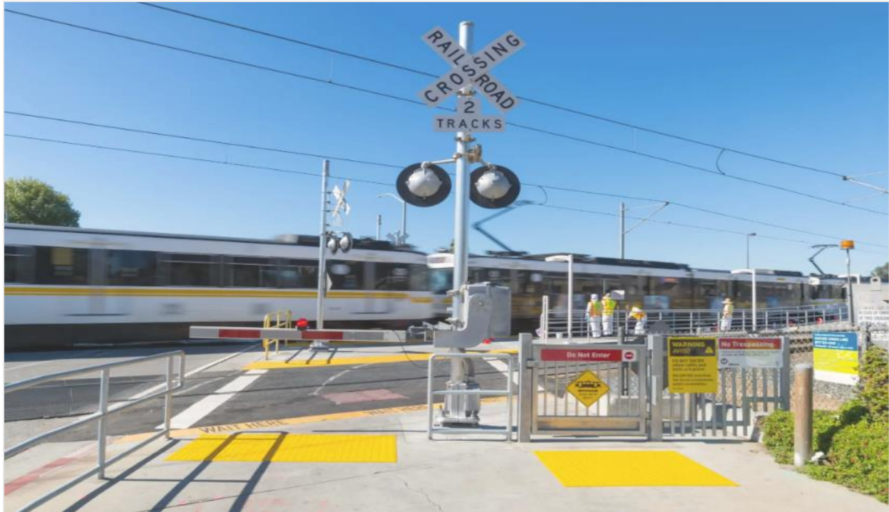
Figure 6-23: Example of Detectable Warning Surfaces and Pedestrian Crossing Enhancements in Los Angeles, California
