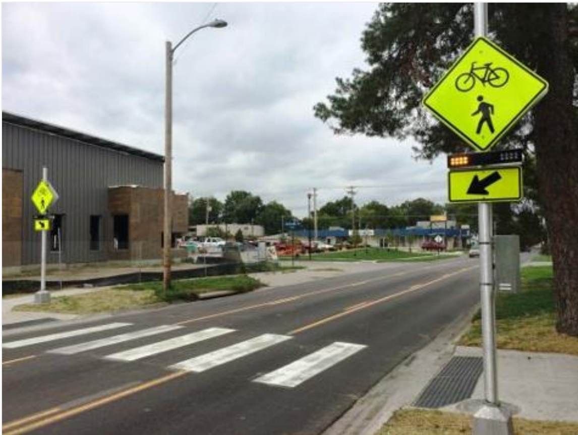
Figure 6-24: Example of Rectangular Rapid Flashing Beacon in the City of Lincoln, NE
