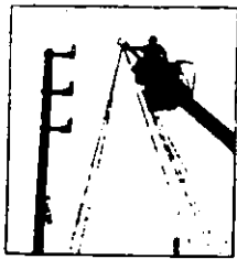
More than 1,000 workers labored to restore electric service.
