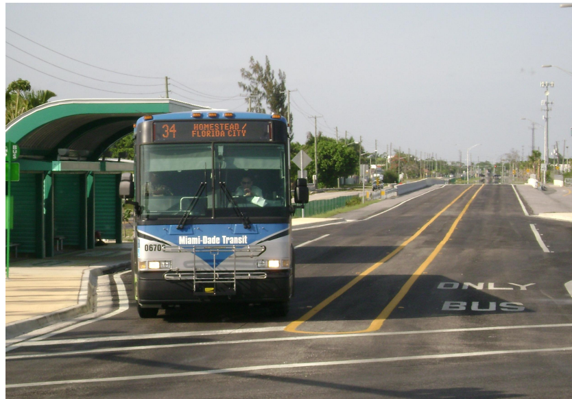
South Dade Busway at SW 296 th Street
