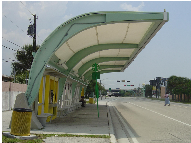
Pedestrian Access to a Busway Station via an Improper Crossing
