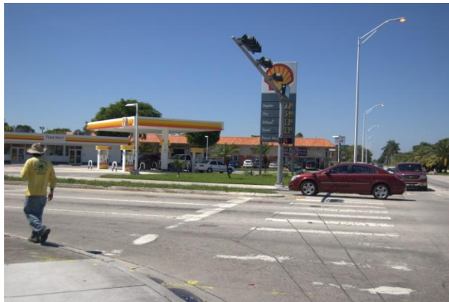
Figure 69: Faded Pedestrian crosswalk markings
