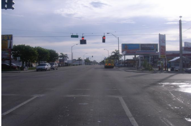
Figure 49: Faded road markings at NW 22 Ave and NW 20 St
