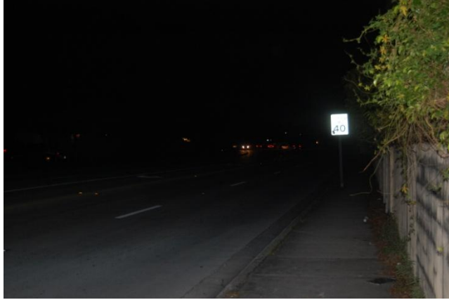
Figure 73: Improper lighting condition
