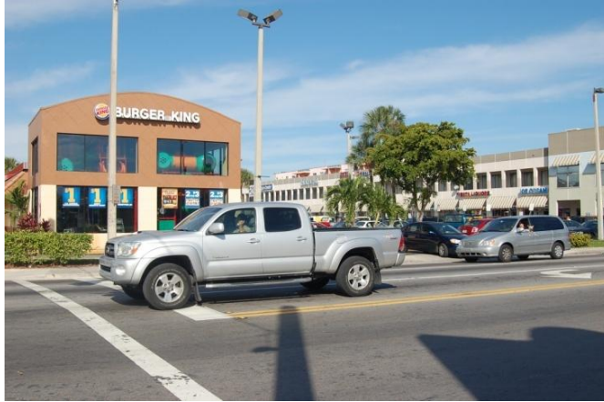
Figure 66: Stop line closer to the pedestrian crosswalk at NW 37 Ave and NW 7St
