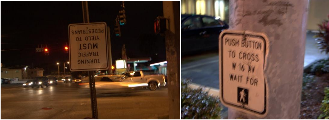
Figure 55: Lacks proper maintenance of infrastructure at NW 22 Ave and NW 20 St
