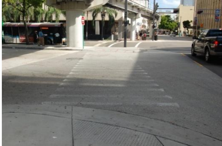
Figure 59: Faded crosswalk at SW 1 Ave and SW 1 St
