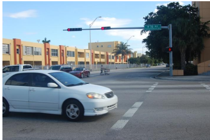
Figure 44: Faded crosswalk and road markings
