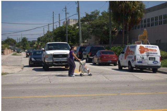
Figure 78: No protection for pedestrians crossing NW 9 ST
