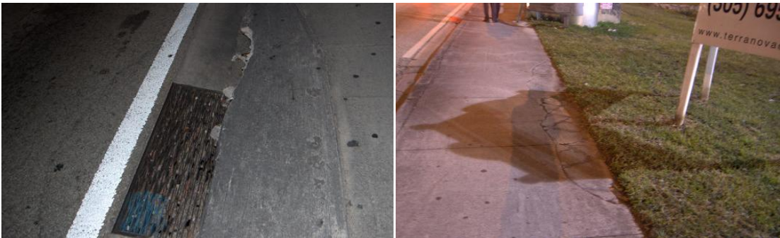
Figure 26: Deteriorating condition of Sidewalk
