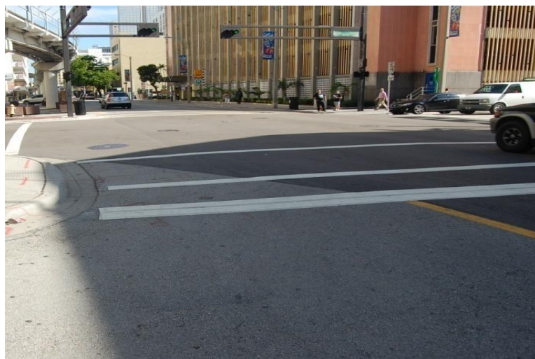
Figure 58: Stop line close to crosswalk at SW 1 Ave and SW 1 St
