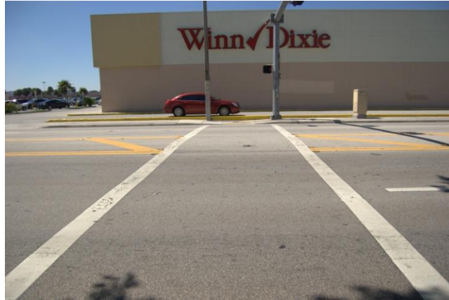
Figure 79: No markings on the crosswalk
