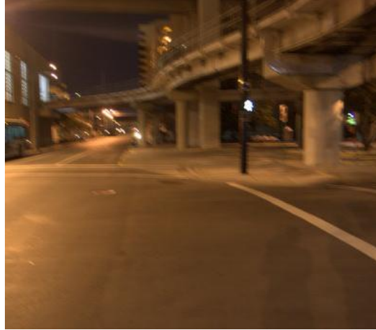
Figure 62: Sidewalks should be expanded to align with road at SW 1 Ave and SW 1 St
