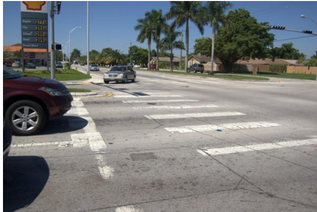
Figure 68: Stop line closer to pedestrian crosswalk
