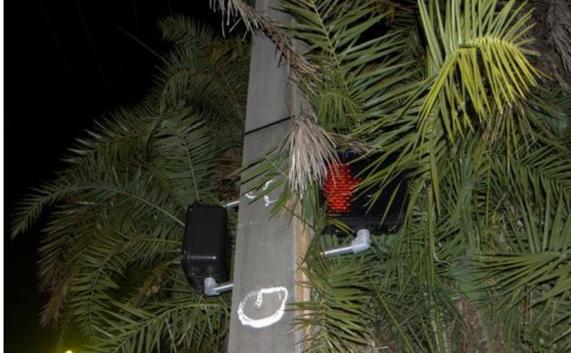
Figure 33: Lacks Maintenance – Branches obstructing view to Pedestrian Signal Head at West Flagler Street and 102 Ave.
