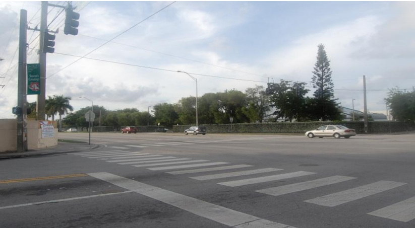
Figure 29: High probability for vehicles to encroach crosswalk – Close to stop line
