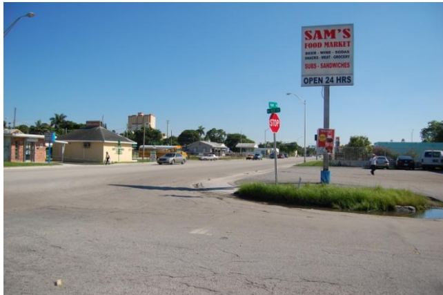
Figure 84: ADA Ramp missing at one corner of NW 83 ST
