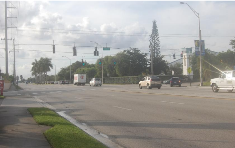
Figure 27: Wide Intersection at West Flagler Street and 102 Ave.
