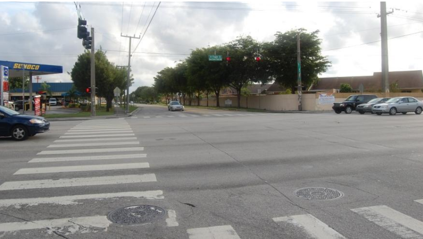
Figure 28: Faded Crosswalk markings
