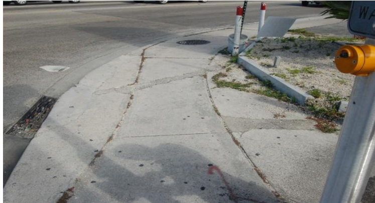
Figure 50: Sidewalks at NW 22 Ave and NW 20 St
