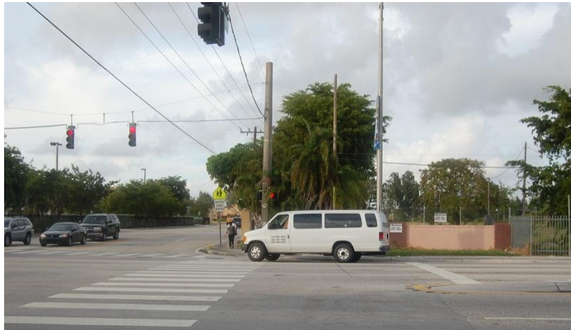
Figure 31: Good distance between crosswalk and stop line.
