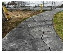
Site Visit at the Hialeah Market Station
