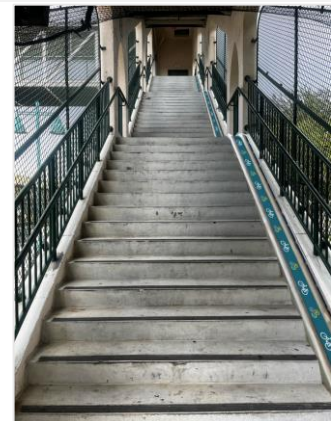
Bicycle Access Ramp
