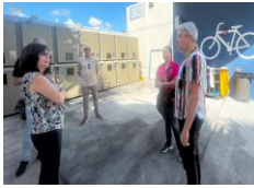
Site Visit at the MIA Station
