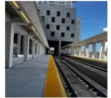
Site Visit at the MiamiCentral Station
