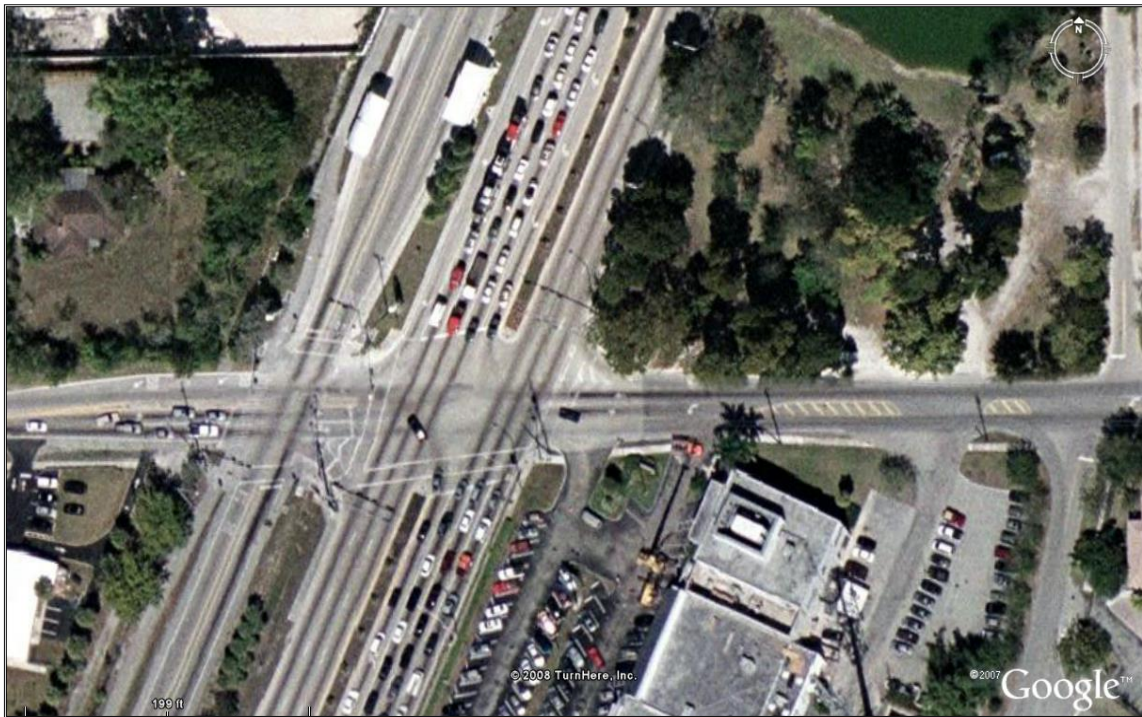
Figure 8.3 Aerial View of SW 112 th Street and US-1 Intersection
