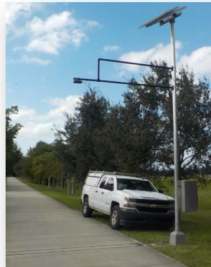
A1A Seaway Drive, Ft. Pierce, St. Lucie County Overhead Infrared with piezo-electric sensors 2023 Avg. Daily Users: 113* ( dual site )
