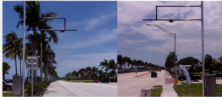
A1A Seaway Drive, Ft. Pierce, St. Lucie County Overhead Infrared with piezo-electric sensors 2023 Avg. Daily Users: 113* ( dual site )
