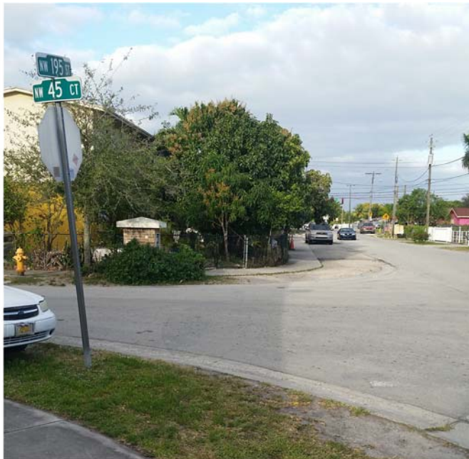
Missing curb ramps and pavement markings
