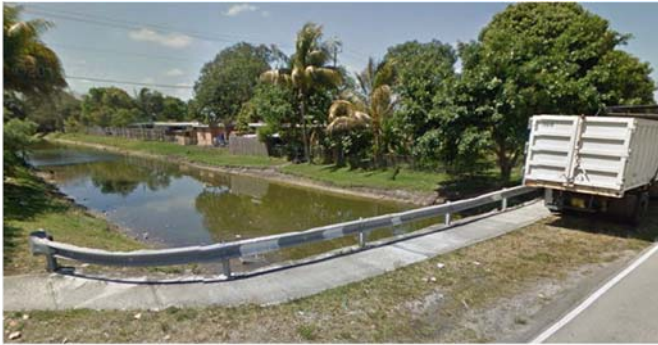
Missing pedestrian railing along canal
