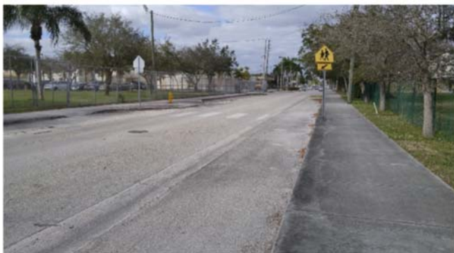
No sidewalk connection to crosswalk
