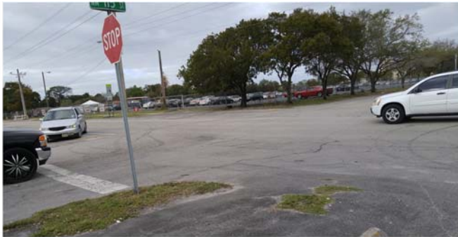
Missing crosswalks and curb ramps
