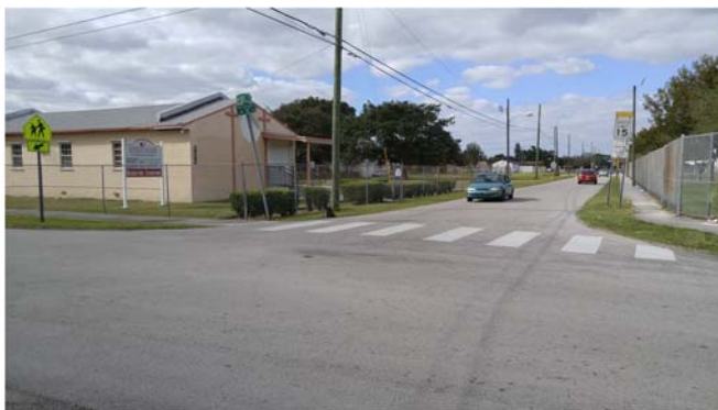
No sidewalk connection to crosswalk
