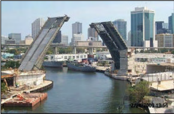
NW 5 th Avenue bridge construction
