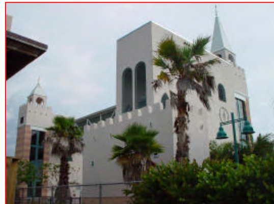
- Ona Locka Tri-Rail Station -
