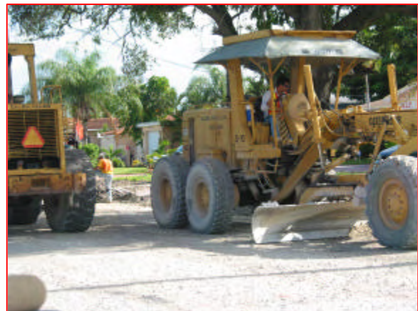
- Road reconstruction work -
