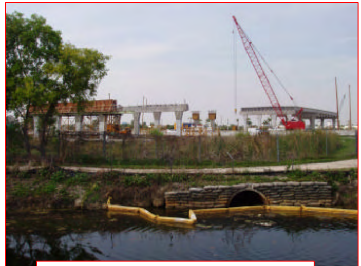
- 97 Avenue Bridge over SR-836 -
