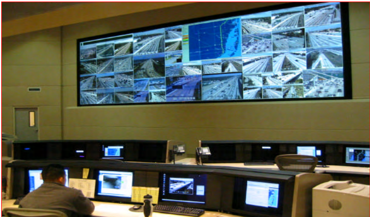
Monitoring Traffic at the Transportation Management Center
