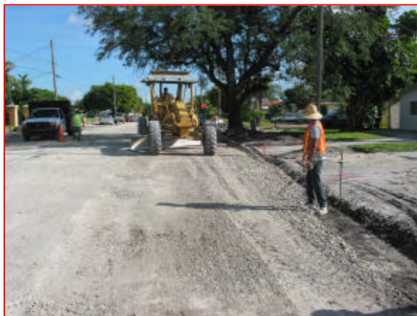
- Road reconstruction in Hialeah -
