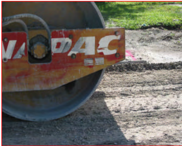
- Private Sector Road improvements -
