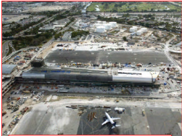
- MIA South Terminal Construction -
