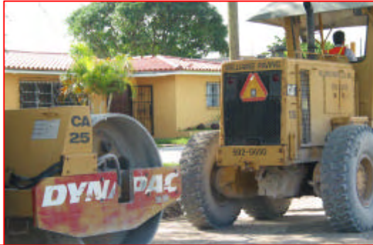
- Roadway Reconstruction Improvement -
