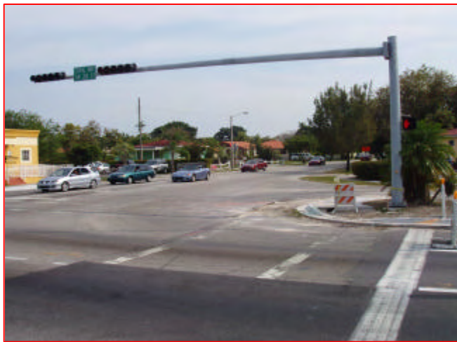
- Installation of Traffic Control Devices -
