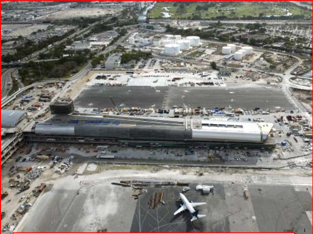
- MIA South Terminal Construction -
