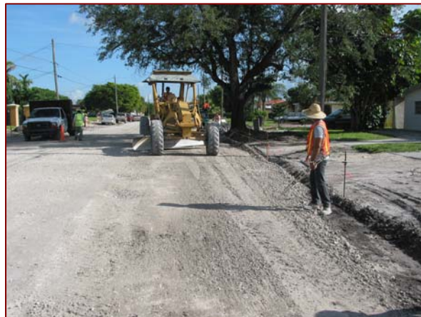
- Road reconstruction in Hialeah -
