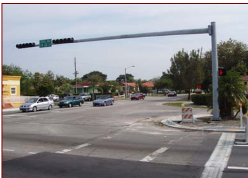
- Installation of Traffic Control Devices -
