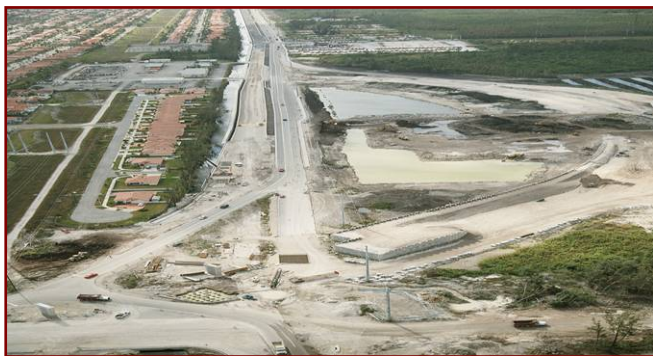
- Extension Project under Construction -
