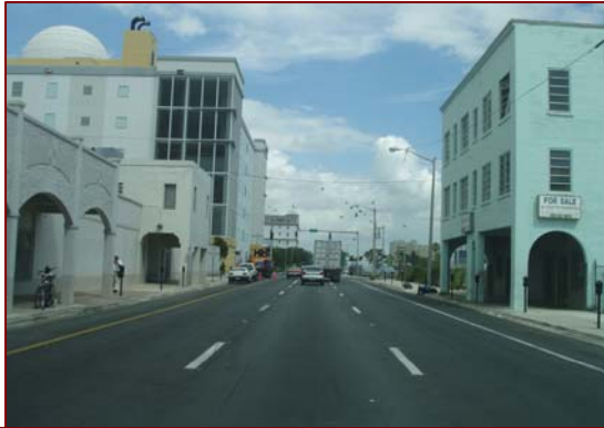
NE 2 nd Avenue Resurfacing
