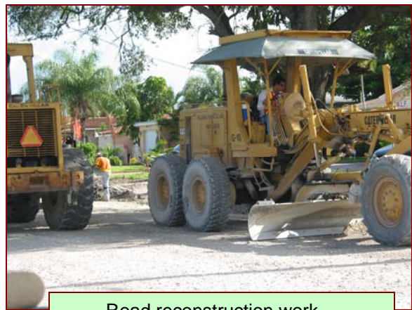
- Road reconstruction work -
