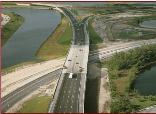
- SR 836 to the HEFT Completed -
