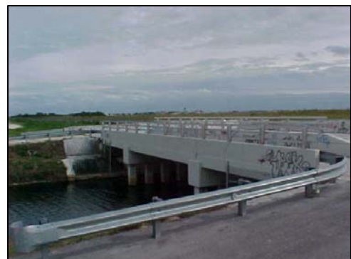
SW 120 St Bridge over Black Creek Canal
