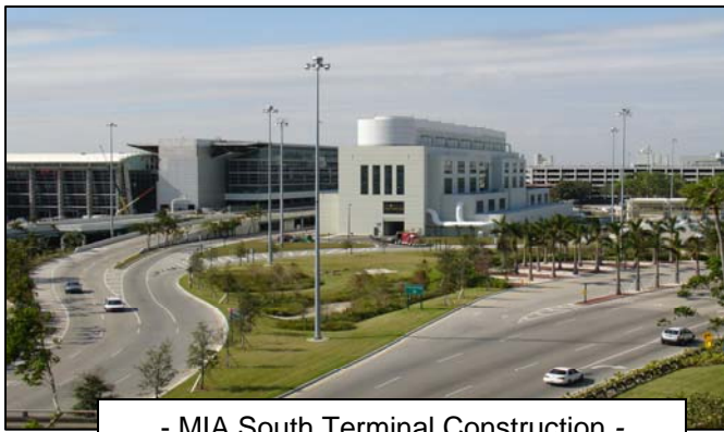
- MIA South Terminal Construction -
