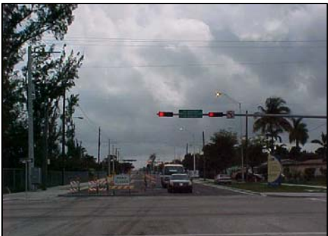
Roadway resurfacing work
