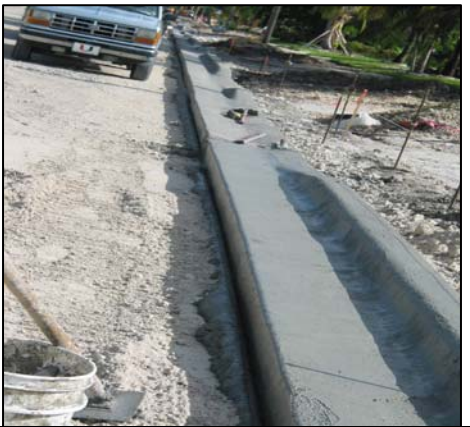
Roadway Curb work
