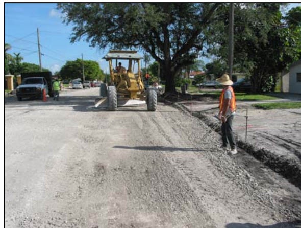
- Road reconstruction in Hialeah -
