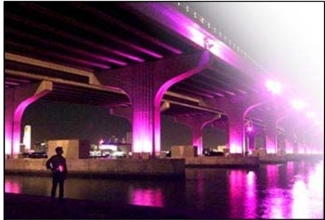
- Port's Access Bridge at night -
