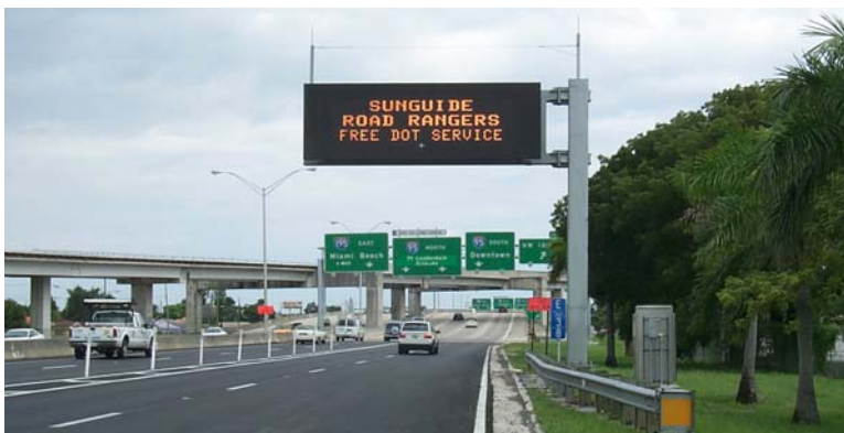
Intelligent Transportation System dynamic message sign.
