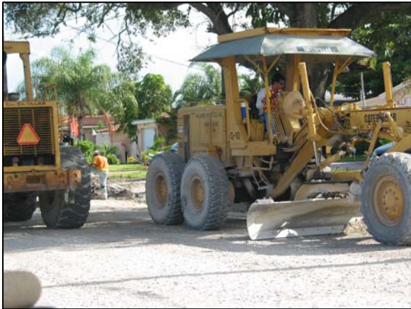
- Road reconstruction work -
