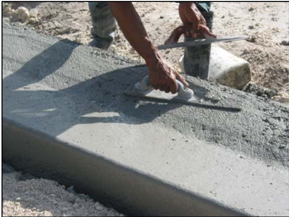
- Road reconstruction work -
