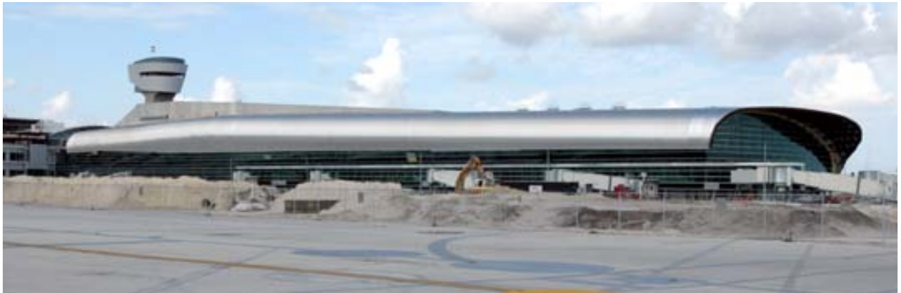
Miami International Airport’s new South Terminal under construction.
