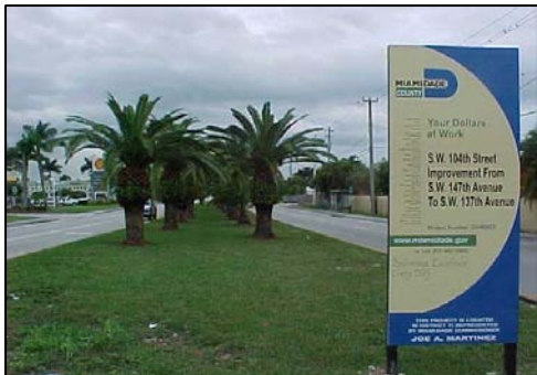
SW 104 Street Improvements
