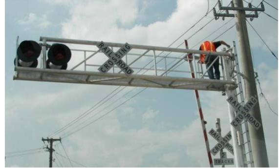
Railroad crossing signal inspection
