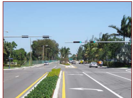
NW 97 Avenue Resurfacing Work
