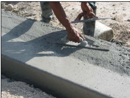
Road reconstruction work
