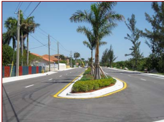
NW 32 Avenue Resurfacing Improvements
