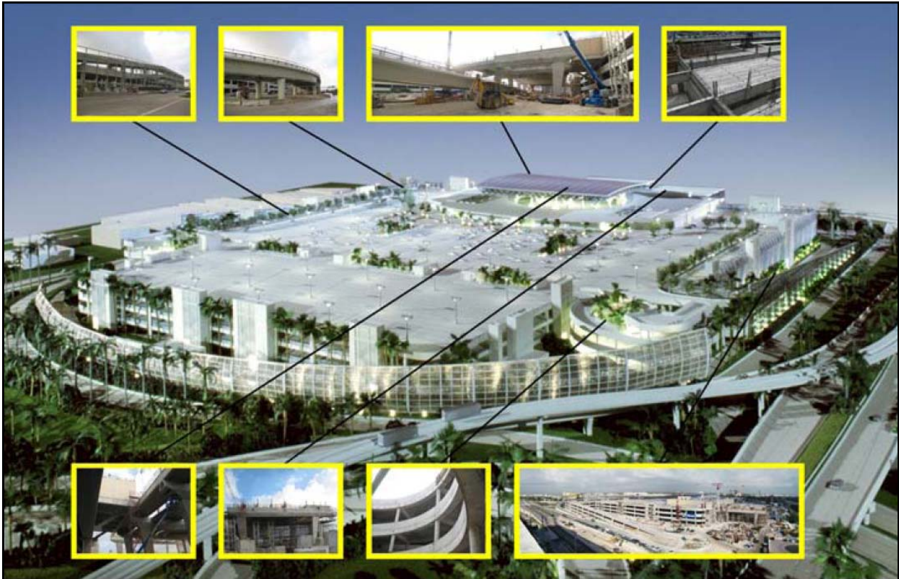
Miami Intermodal Center/Rental Car Facility Presently Under Construction
