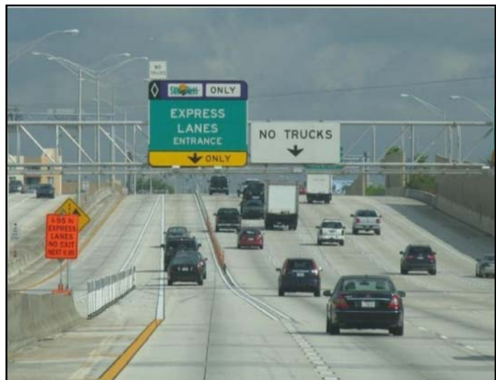
View of the I-95 Express Lanes in the Northbound Direction
