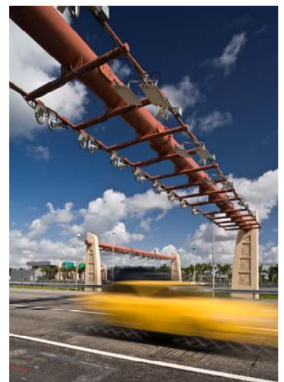
View of typical ORT gantry
