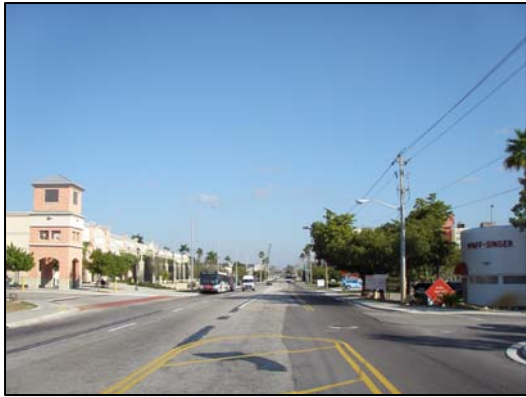
NE 15 th Avenue from 163 to 170 Street
