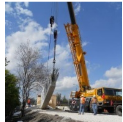
SR 924 ORT Gantry construction.
