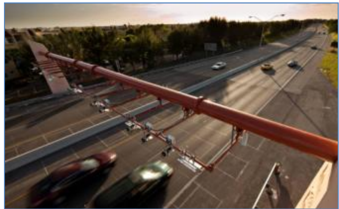
View of Typical ORT Mainline Gantry
