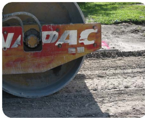
Private Sector Road Improvements
