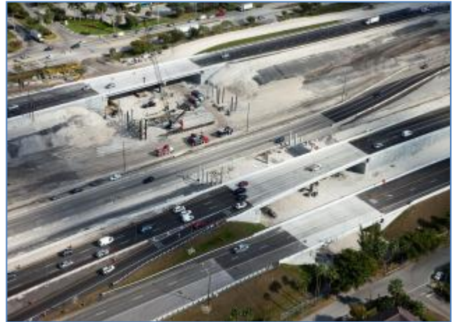
SR 836 EB CD Roads & Bridges over 87 th Ave.
