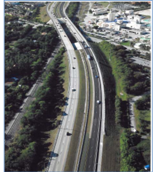
SR 874 SB at 87 th Ave and CXS Railroad
