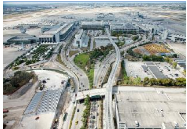
Central Blvd. Looking West
