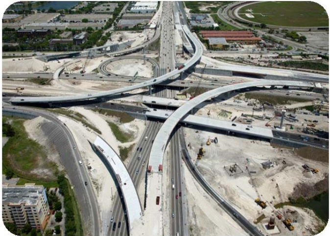
SR 826 / SR 836 Interchange
