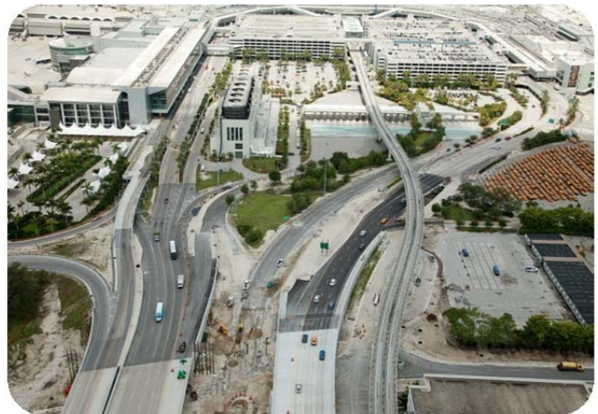
Central Blvd. at Perimeter Road Bridge
