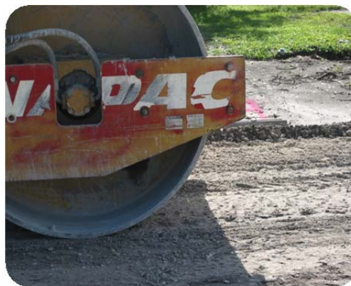
Private Sector Road Improvements
