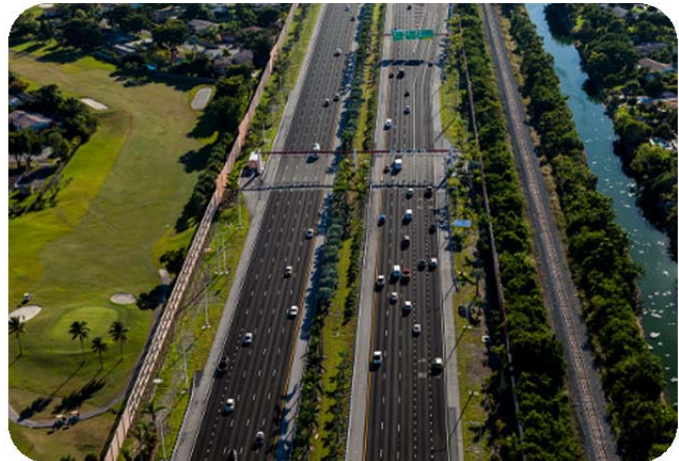
SR 874 / Killian Parkway Interchange
