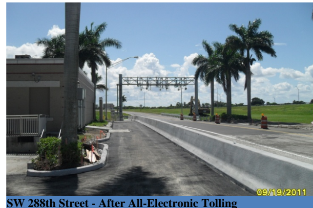
SW 288th Street - After All-Electronic Tolling
