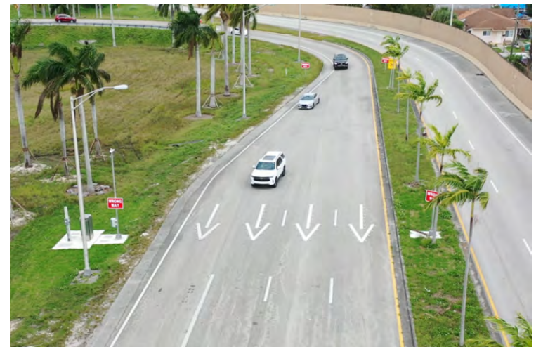
Wrong Way Driving Improvements at Flagler Street (Phase 1)
