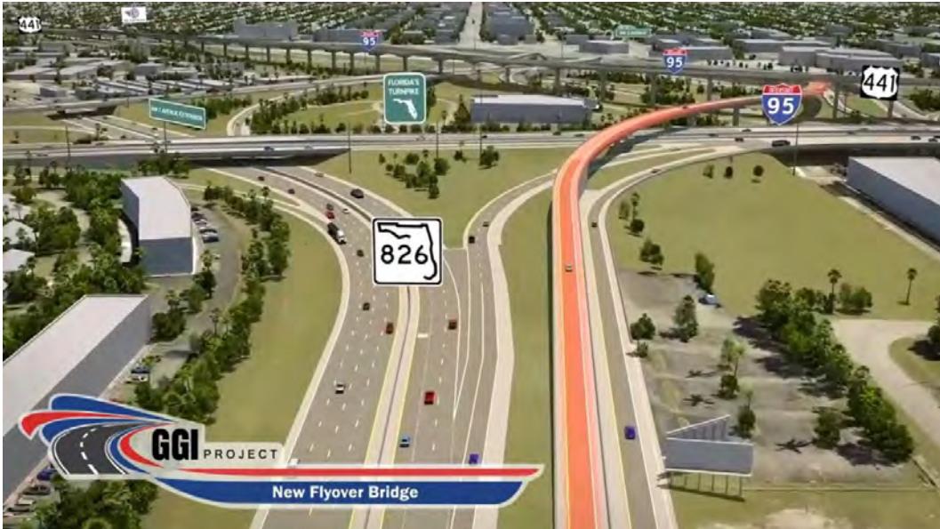
Golden Glades New Flyover Bridge
