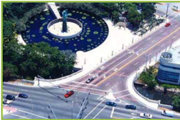
Meridian Avenue Bridge, Miami Beach
