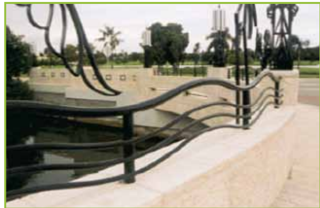
Meridian Avenue Bridge
