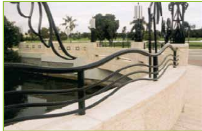
Meridian Avenue Bridge
