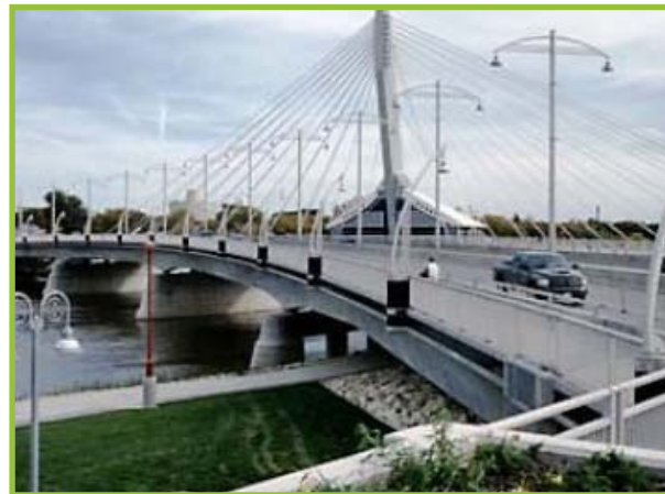
Creation of Iconic Bridges - Winnipeg Manitoba, Canada
