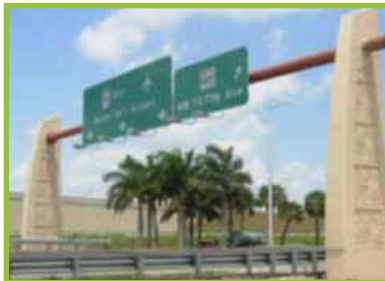
MDX Sign Structure
