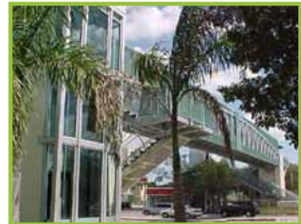
Douglas Road Pedestrian Overpass
