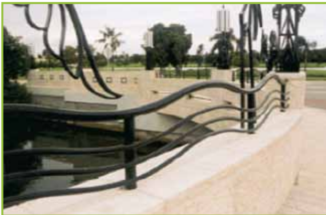
Meridian Avenue Bridge
