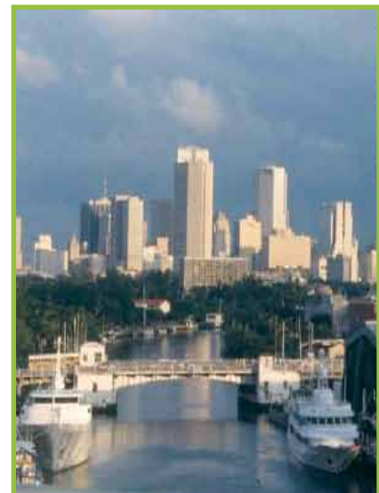
Miami River Bridges
