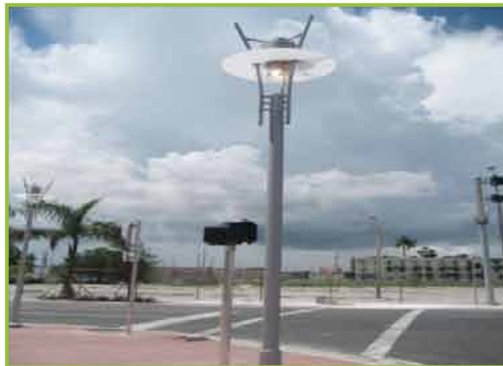
PAC Typical Lighting Fixture - Miami, Florida
