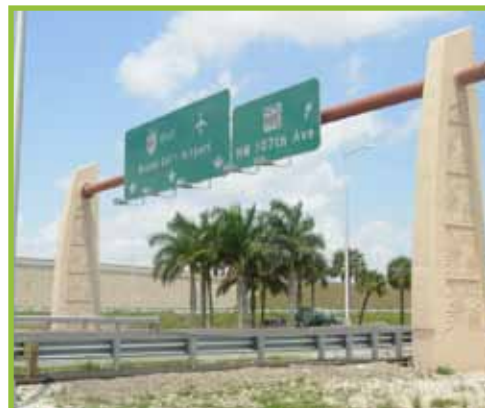
MDX Overhead Signage Structure
