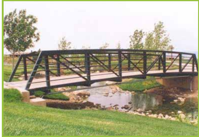
Stream and wildlife crossing, Henderson, Nevada
