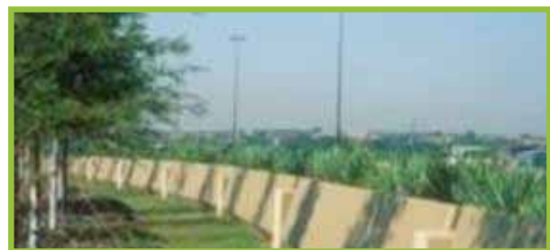
Dual concrete guardrails used as a planting bed, North Central Expressway, Dallas, TX
