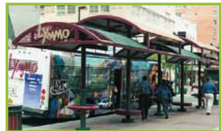
LYNX bus shelter, Orlando, FL
