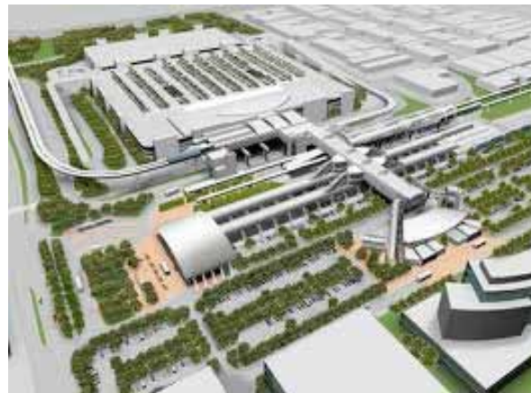
Metrorail Station at the Miami Intermodal Center
