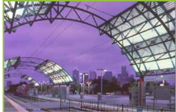
Dallas Area Rapid Transit – Cedars Station, Dallas, Texas
