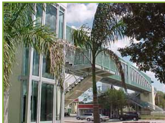
Pedestrian Bridge over US-1 at Douglas Road
