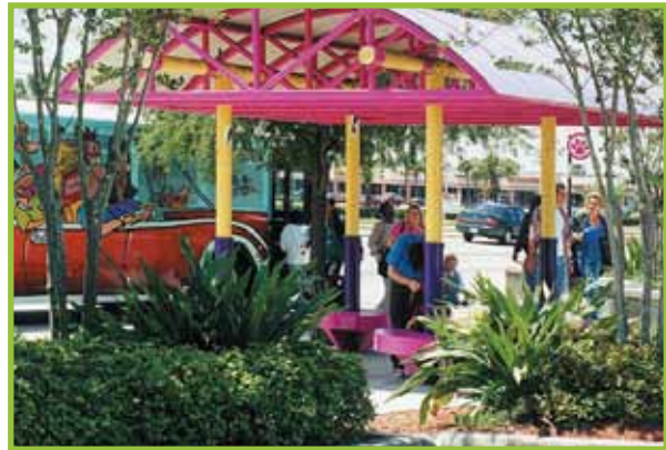
LYNX bus shelter, Orlando, Florida
