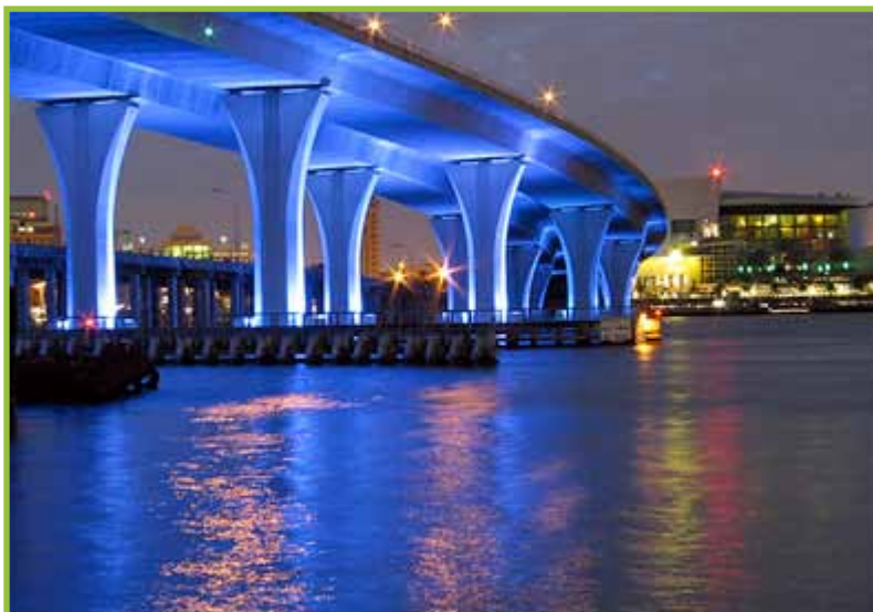
Port of Miami bridge
