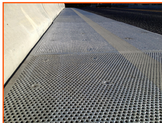
Anti-slip metal plates over shoulder on Hillsboro Inlet bridge in Broward County, FL
