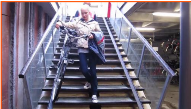
Rails along stairs in multi-level transit station in the Netherlands allows for easier mobility for passengers with bicycles
