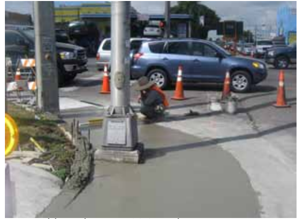
Mountable curb at NW 20 St and NW 17 Ave.
