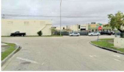
VA 3 rd COURT - BEFORE
